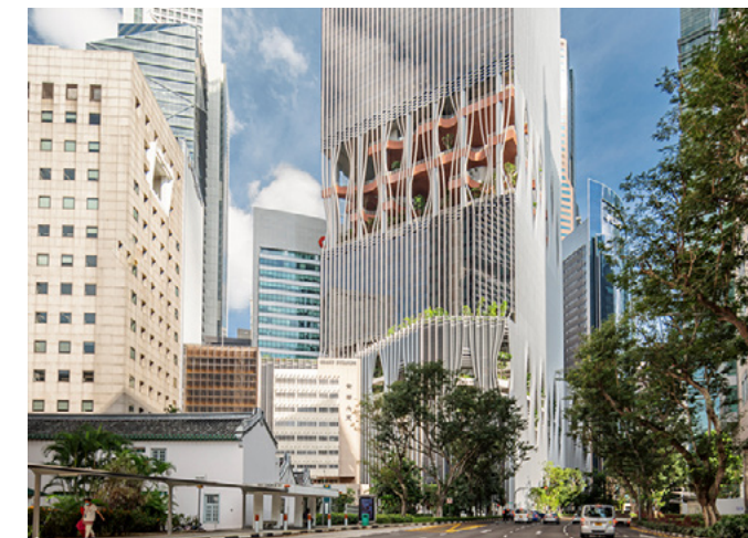
CapitaSpring's facade is designed to showcase the building's green terraces and communal spaces, while maximising daylight and minimising heat gain. Image by CapitaLand
